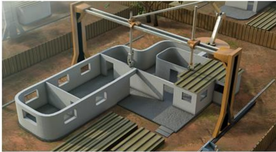
Figure 5: The printer behind “Contour Crafting”.
